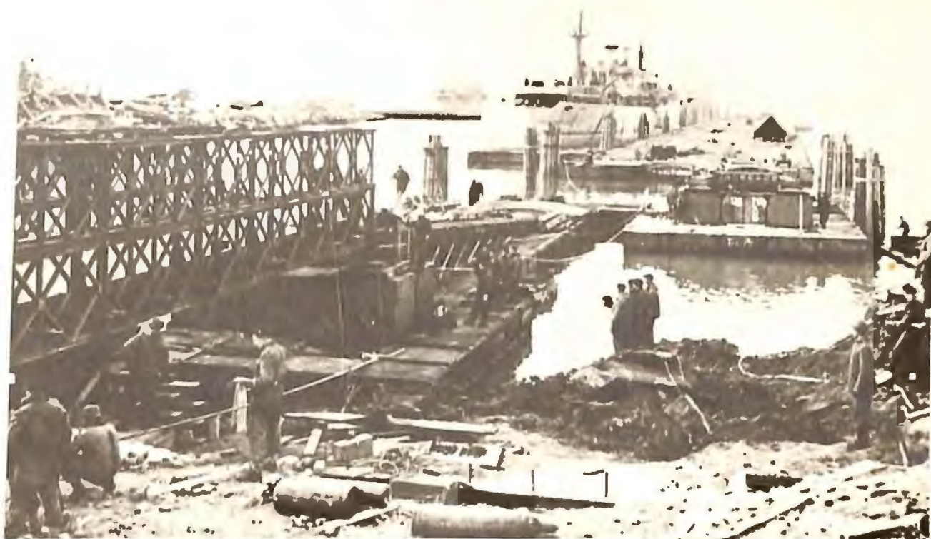
SHORE END SHOWING BAILEY BRIDGES NAVAL PONTOON PROJECT- LE HAVRE - FRANCE
