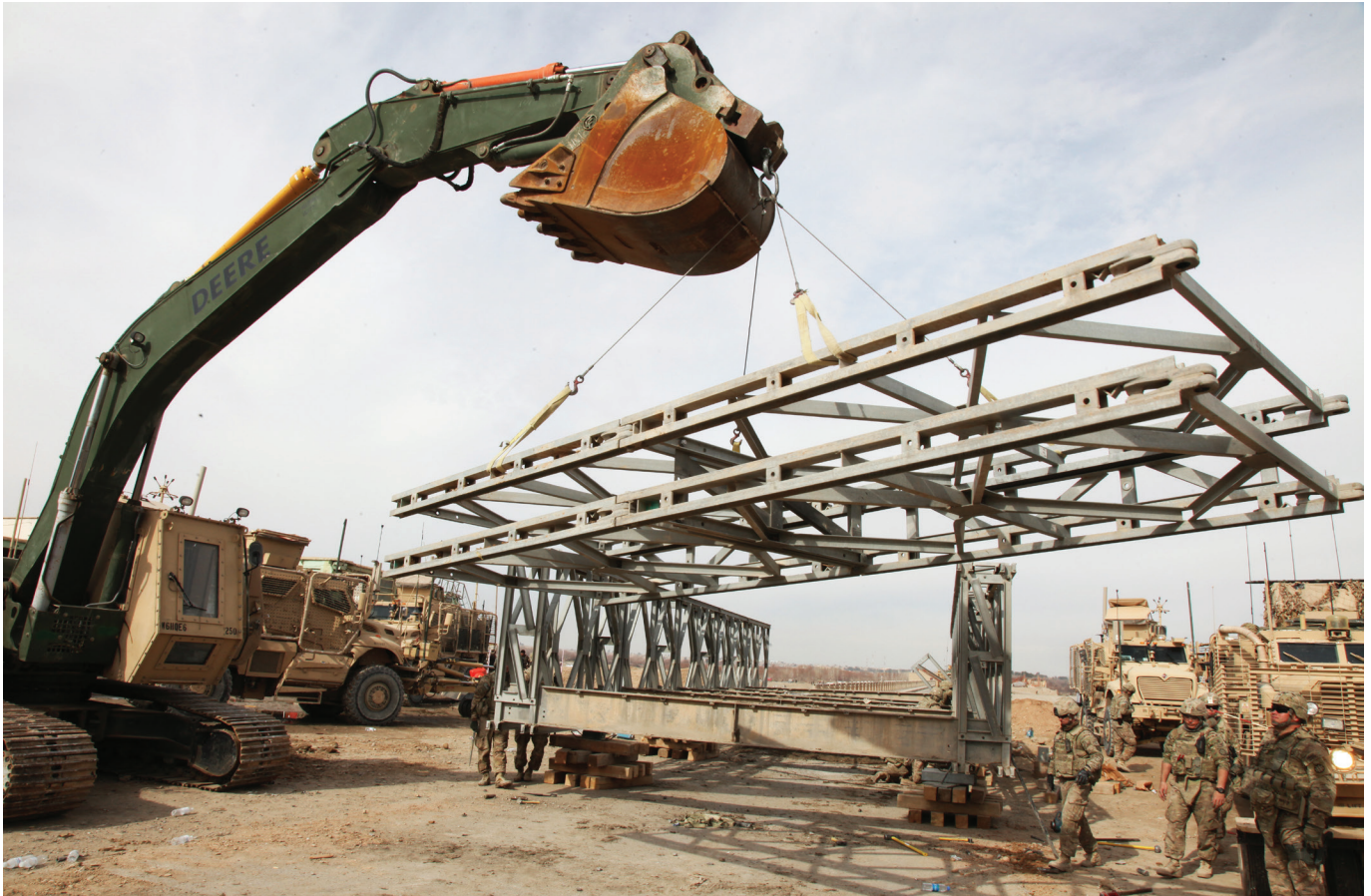
Soldiers of the 1438th Multi-Role Bridge Company, Missouri National Guard, disassemble an over bridge in Gereshk, Helmand province, Afghanistan. The over bridge was a replacement for a bridge that had been damaged during an insurgent attack. The Theater Engineer Brigade sustainment cell disassembled U.S. and NATO Acrow Bridge sets so that they could be replaced by more permanent structures that Afghan units will maintain. (Photo by Cpl. George Huley)
