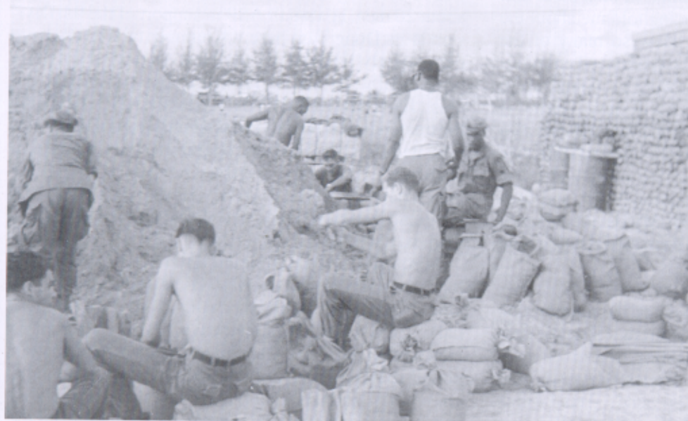
□ To construct a new bunker after the April 1968 rocket attack on Vung Tau, soldiers made sandbags after completing their daily ASP work. Vietnamese laborers then used the sandbags to build the bunker.
