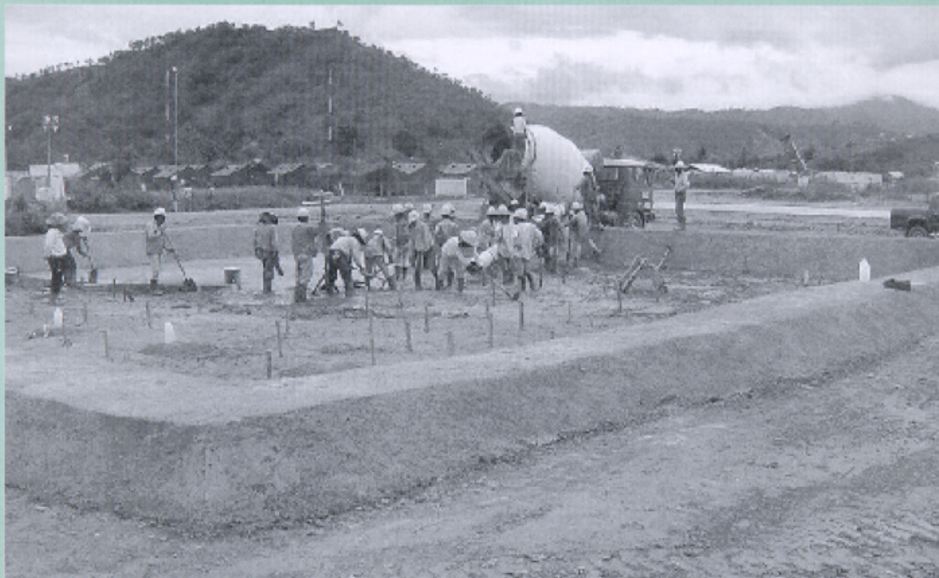
□ The LOGCAP contractor employed dozens of local nationals. Here, they assist in pouring concrete for the fuel point.
