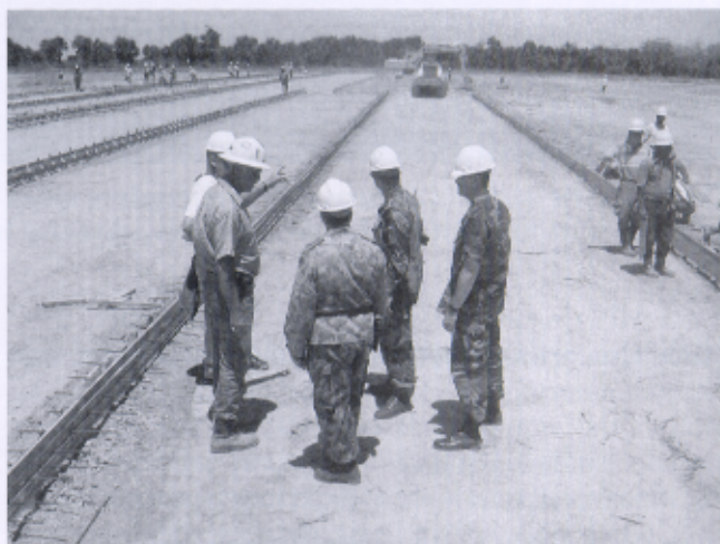
□ Army and contractor personnel survey the construction site for the helipads at Comoro Airfield in Dili. The LOGCAP engineering subcontractor, Fluor-Daniels, had to create a cement production facility from scratch in order to build the helipads.
