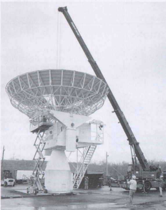
□ Tobyhanna Army Depot employees, assisted by Defense Distribution Depot-Tobyhanna's crane crew, attach an OE-222/G antenna dish reflector to reflector arms.
