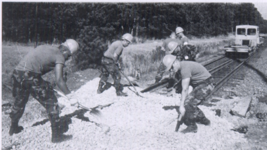
□ Soldiers of the 1205th Transportation Railway Service Unit spread rock ballast while repairing a rail line at Sunny Point.
